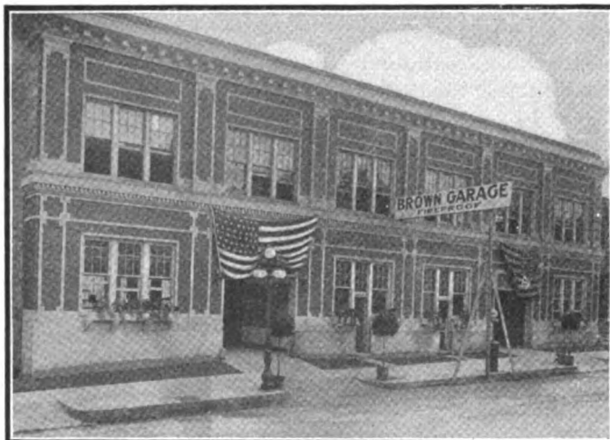
Brown Garage in Des Moines, Ia., which is rendered attractive by means which unfortunately are unusual in garage construction
